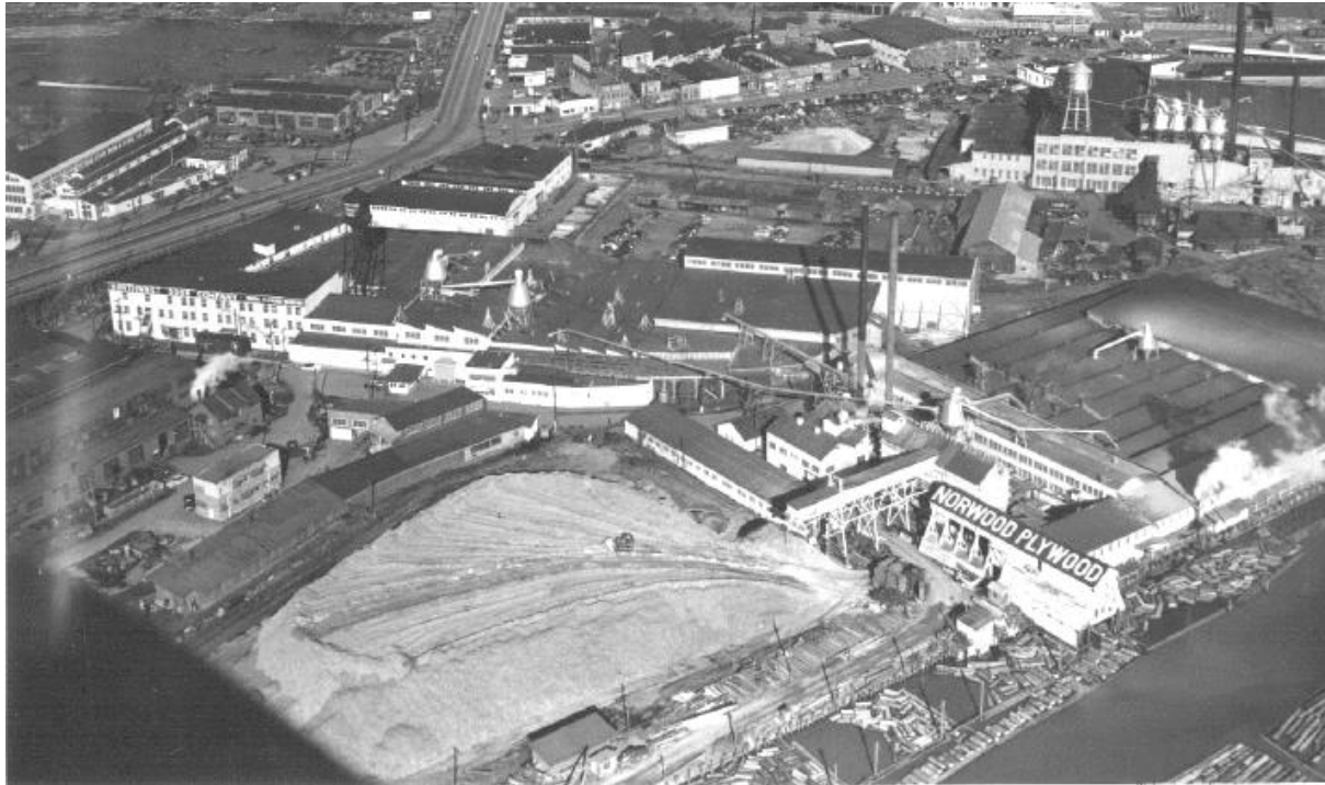
Parcel 94 (1948) - View of the Norwood Plywood and Door Operations
